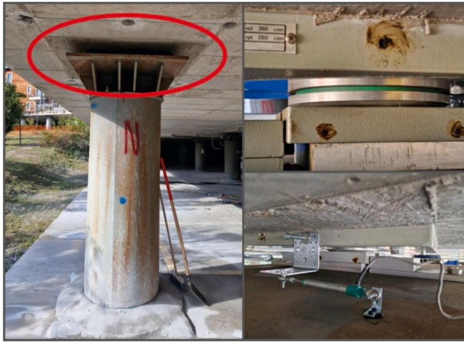
Fig. 6. Isolation bearing placed on the top of the steel column.
