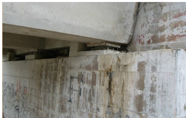
Figure 3.8. Shear keys and bearings
