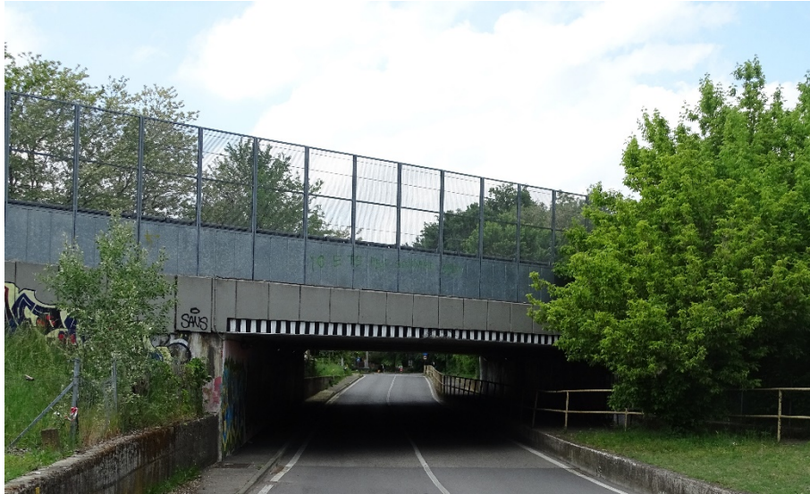
Figure 9 - Example of R.C. bridge of the MSE portfolio
