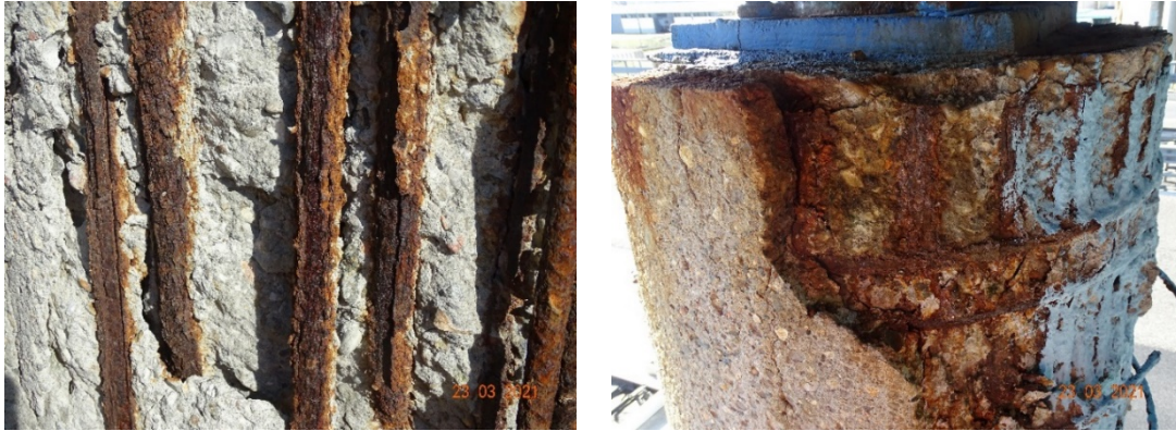
Figure 23 - Corroded reinforcement
