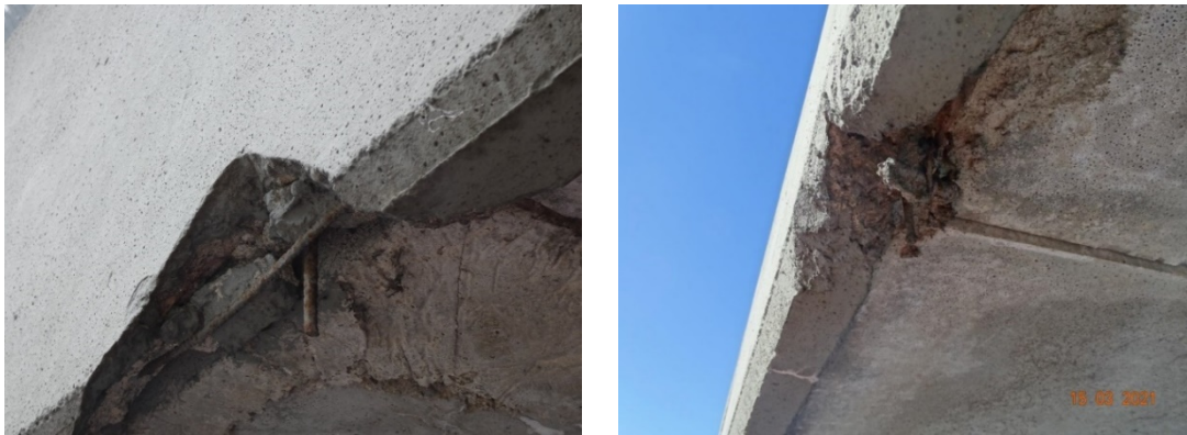
Figure 39 - Impact damage
