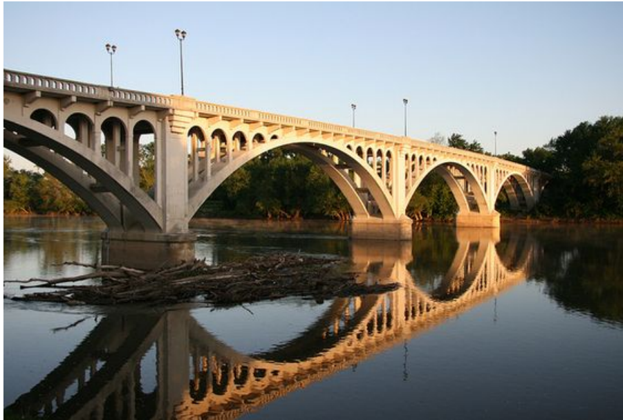
Figure 4 - Reinforced concrete arch bridge example
