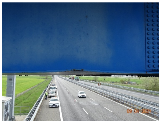
Figure 14 - Flange deformation
