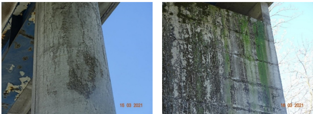
Figure 20 - Deteriorated concrete
