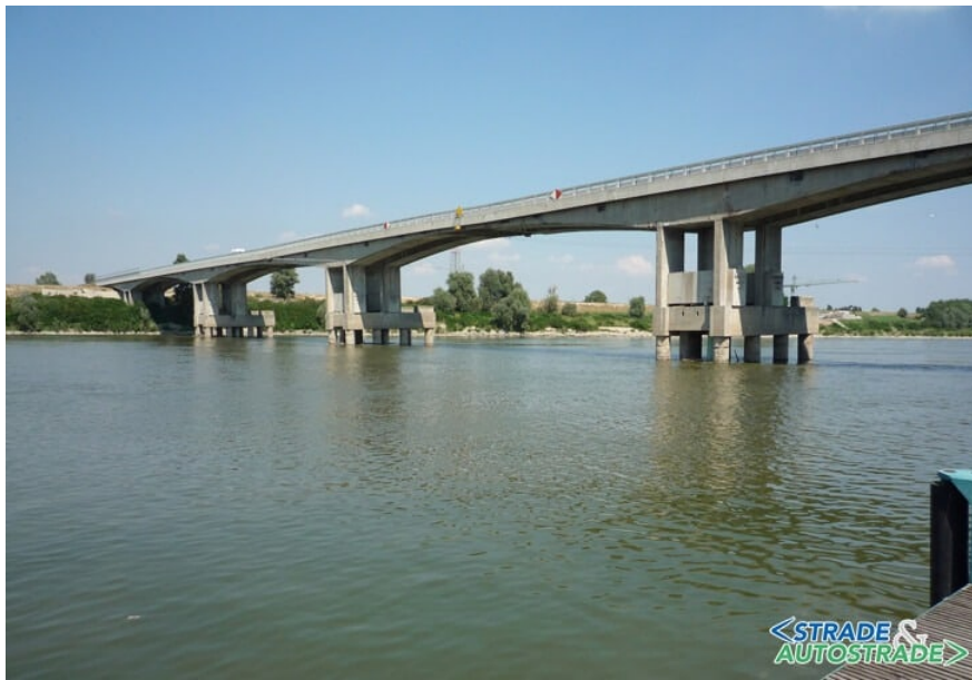
Figure 6 - Gerber bridge example
