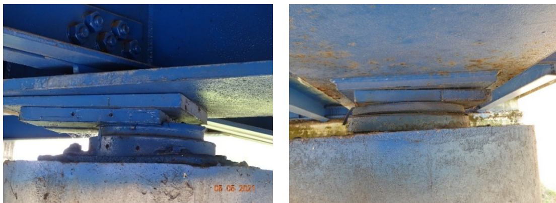
Figure 34 - Incorrect presetting
