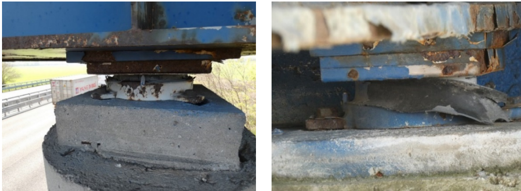
Figure 36 - Neoprene/Teflon deterioration
