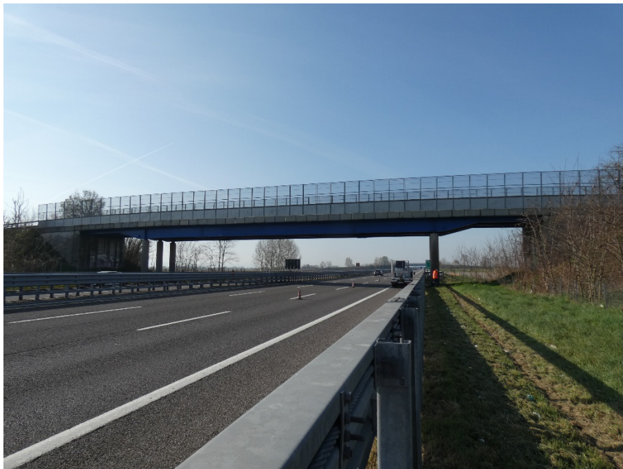
Figure 10 - Example of mixed R.C. and steel bridge of the MSE portfolio
