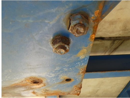
Figure 13 - Bolting defect
