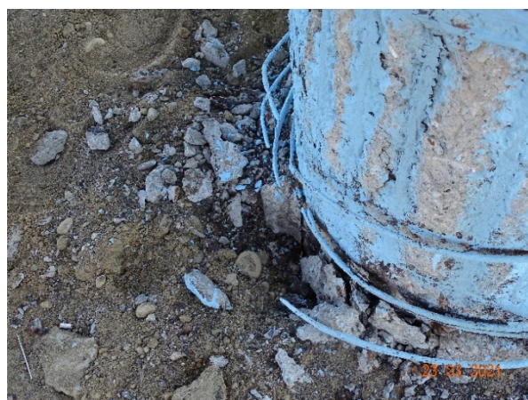
Figure 30 - Broken stirrups
