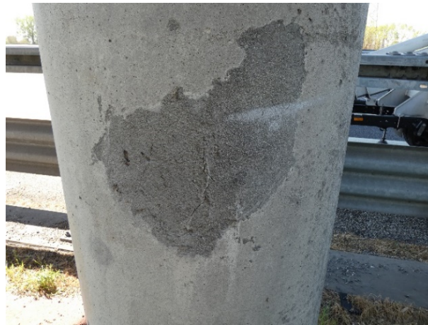
Figure 26 - Deteriorated reparations
