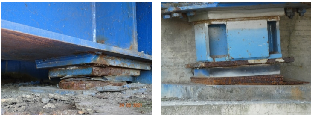
Figure 31 - Deformed baseplate
