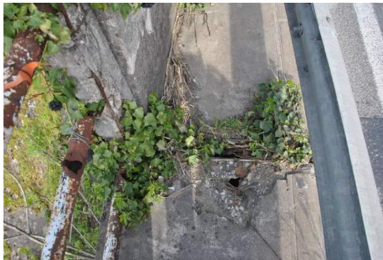
Figure 44 - Permeable or absent flashing (Adopted from Annex C of the Italian guidelines)
