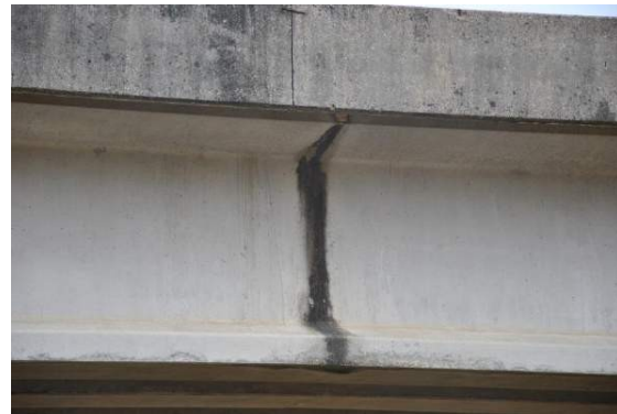
Figure 44 - Permeable or absent flashing (Adopted from Annex C of the Italian guidelines)
