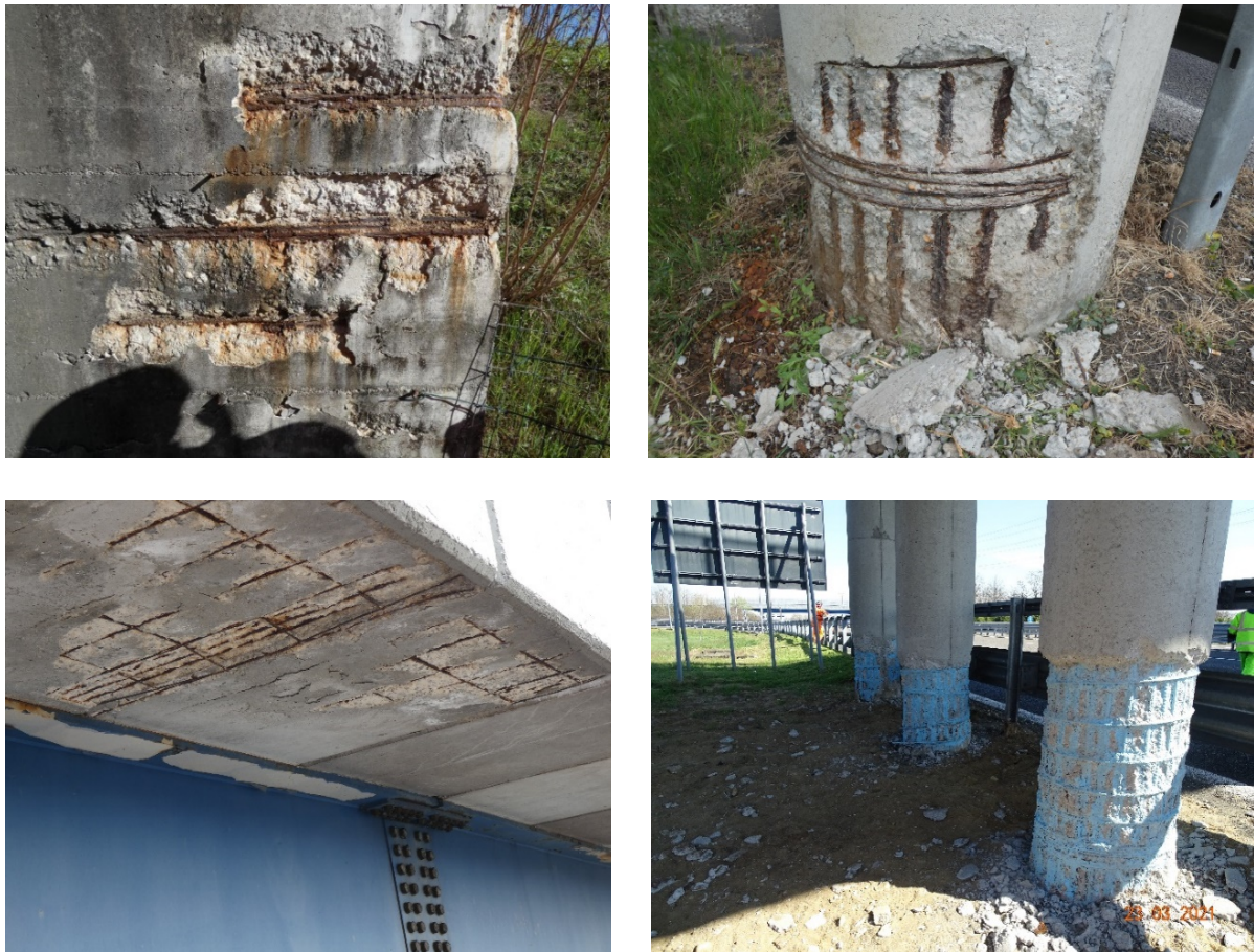
Figure 22 - Concrete spalling
