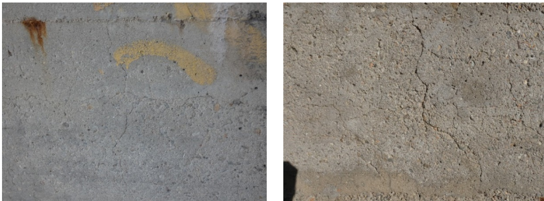
Figure 24 - Minor cracks
