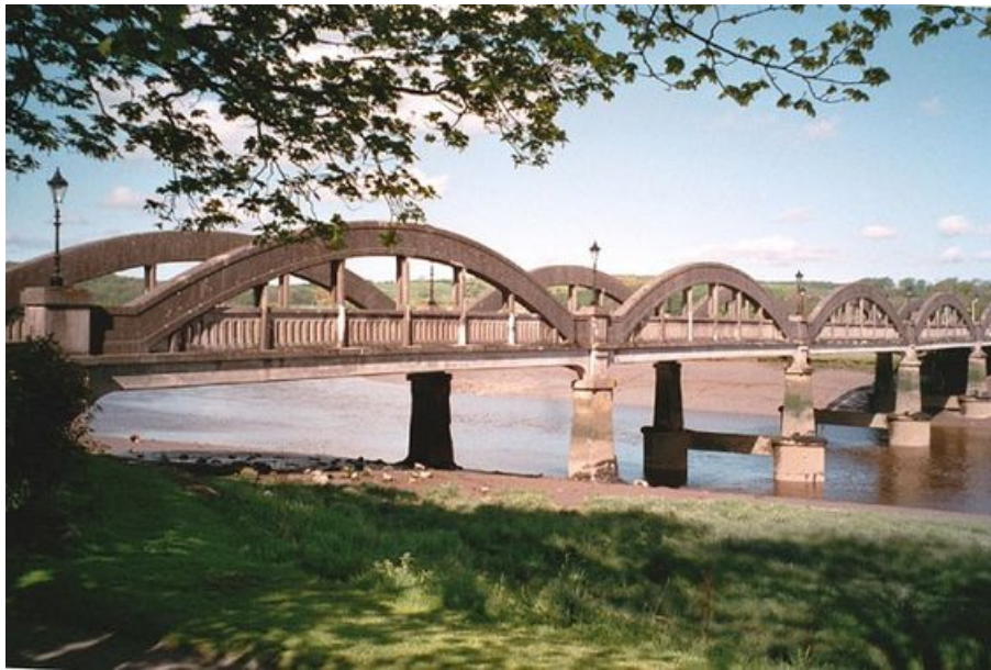
Figure 5 - Reinforced concrete tied-arch bridge example
