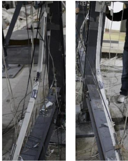
Figure 6: Plastic deformation of the bracing members under shake table excitation. (Goggins et al. 2021)
